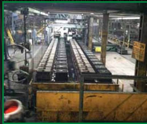
Molds are indexed to shakeout with the Roberts Sinto mold handling system.
