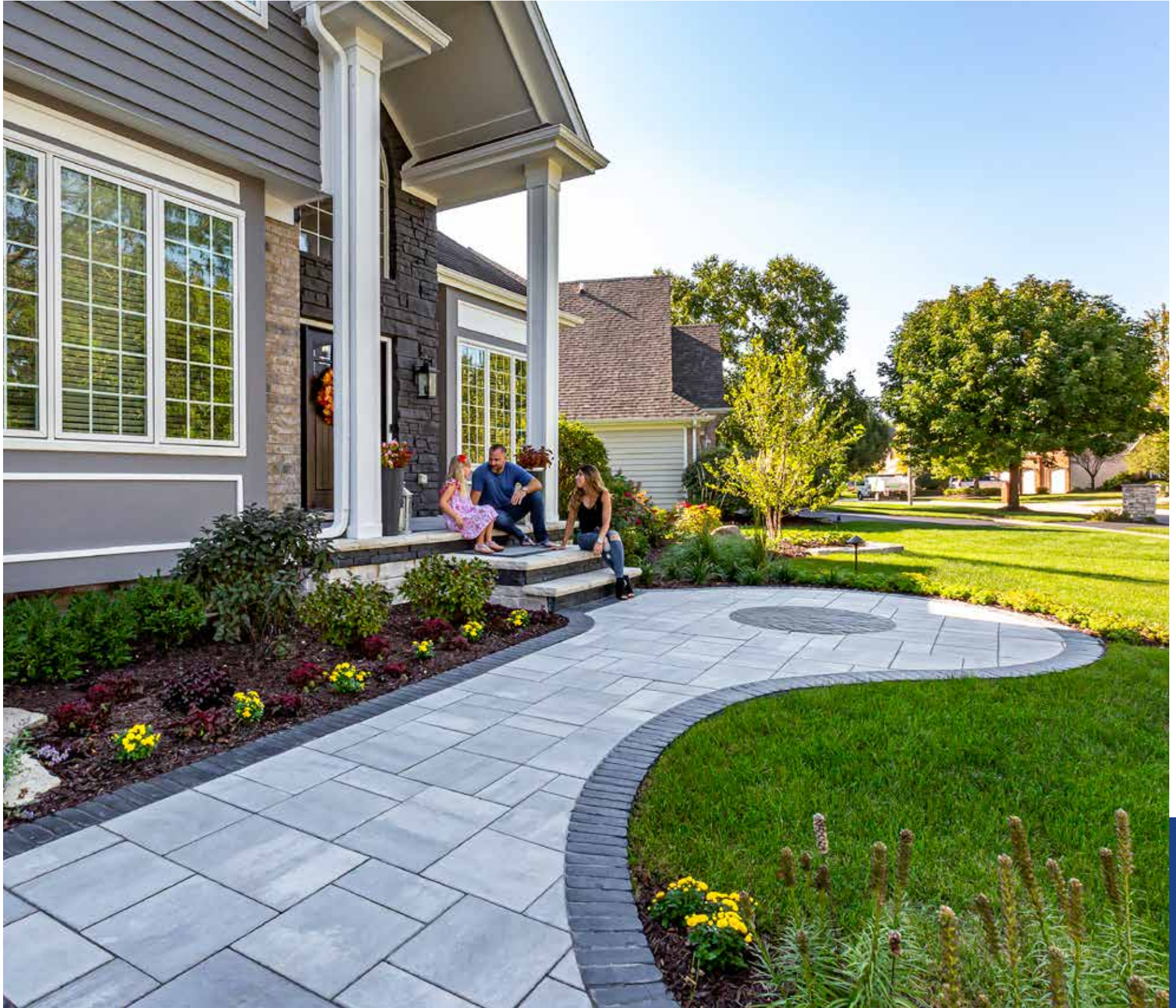
Pavers: Beacon Hill™ Smooth (Granite Fusion) with Copthorne (Basalt) accents Steps: Copthorne (Basalt) accent fascia with Ledgestone™ (Buff) step treads
